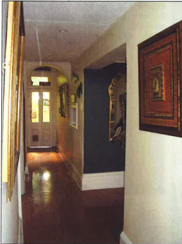
Figure 3.34 The secondary, traverse hall at the junction of the main and rear wing on the ground floor has ripple iron ceiling with simple coving. An arch and side door (to small porch on north western façade) is located at the northern end, adjacent to the kitchen.
