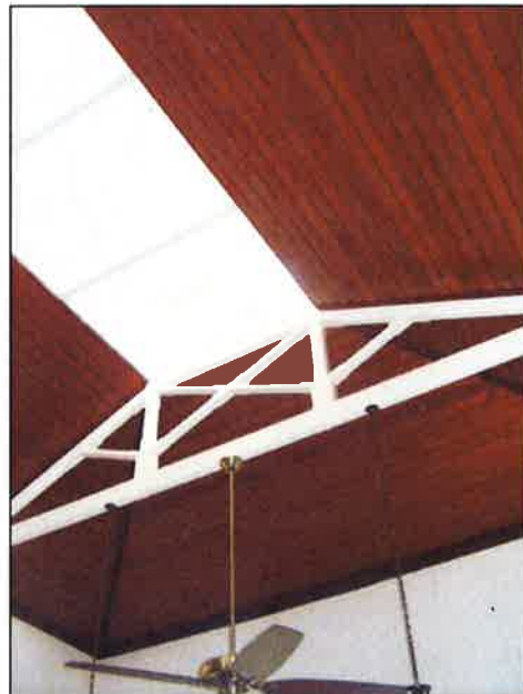
Figure 3.37 The most notable feature of the rear wing is the central, double height space which has timber panelled ceiling, exposed timber trusses and high clerestory windows.
