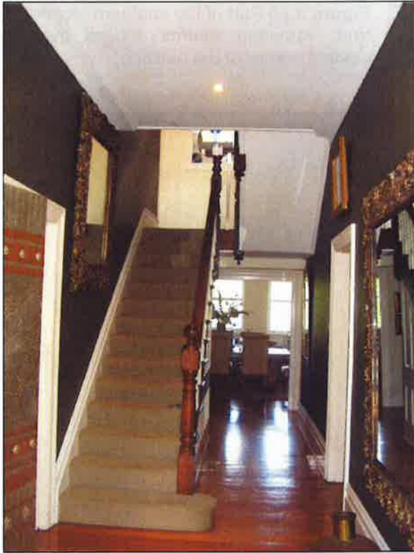
Figure 3.26 The ground floor central entry hall and stair. The interior generally retains timber floor, rendered and set walls and timber joinery. The hall has simple plaster ceiling with deep, flat coving. The hall is bounded by four main rooms and also leads directly into the large ground floor room (former ballroom) on the ground floor. A leaded window on the stair landing remains a feature of the room.
