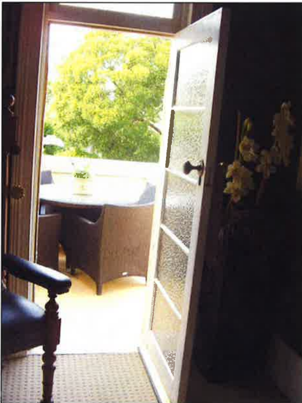
Figure 3.41 A deep window opening on the eastern wall of first floor hallway has been converted into a doorway and accesses the balcony over the front verandah.
