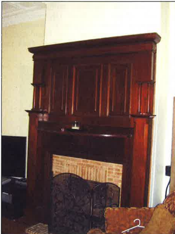
Figure 3.31 The room also retains what is assumed is an original timber fireplace surround, however, the fireplace appears to have been modified.
