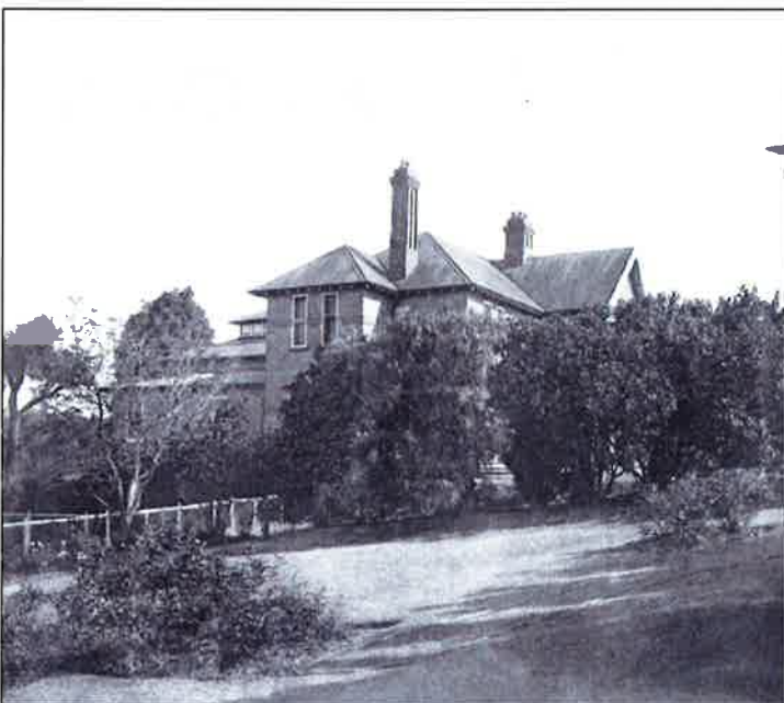
Figure 2.5 Lanosa , 1920. The raised roof and clerestory window over the rear wing are visible.
