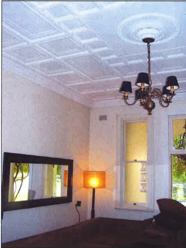
Figure 3.30 The north western room on the ground floor of the main wing retains a high decorative plaster ceiling and original timber joinery. A window has, however, been modified with door added to access the northern verandah.
