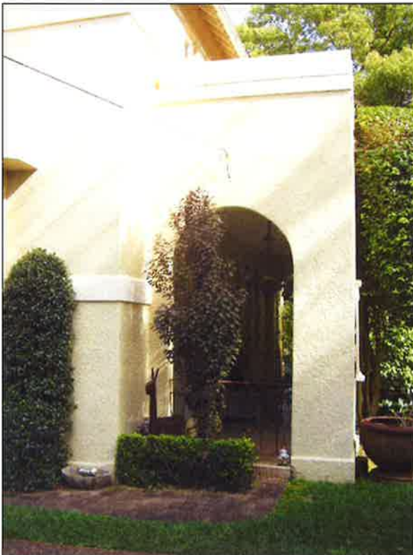
Figure 3.19 A verandah with arched colonnade has also been added to the north eastern façade. Window openings on the ground and first floor appear to have been altered and replaced with doors to access the verandah and open balcony over.
