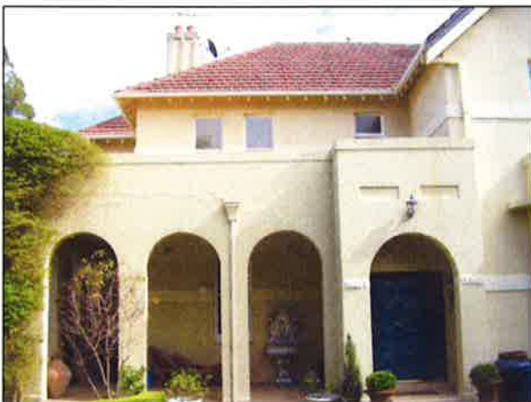
Figure 3.17 The verandah and entry have a solid parapet/ balustrade and open balcony over. The verandah arches are a later addition and reflect the original arched entry (at right). A deeper window opening on the first floor level appears to have been converted into a doorway to access the balcony. The two chimneys also appear to have been altered and height reduced at some stage.
