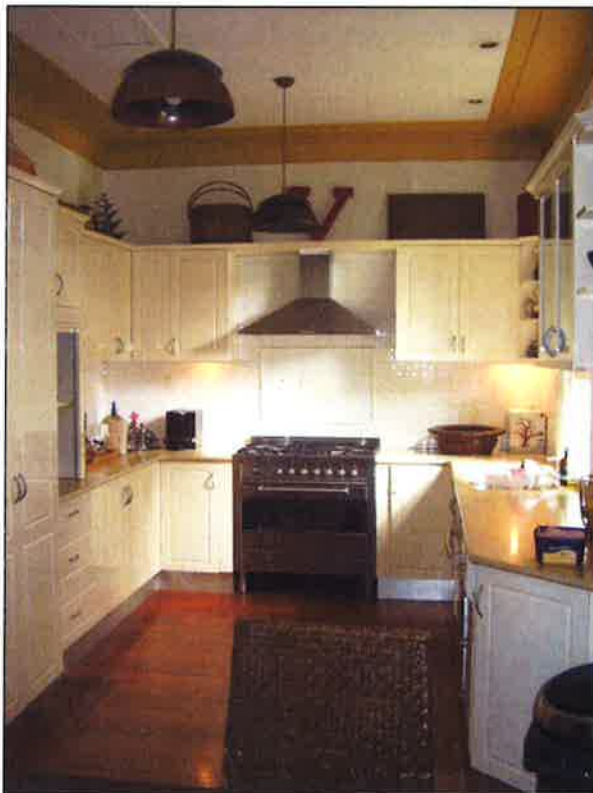
Figure 3.35 The kitchen located on the ground floor and northern side of the rear wing has modern kitchen cabinets, fixtures and fittings and simple plaster ceiling with flat coving (typical of 1930s-1940s which suggests the ceiling was replaced as part of the early 1940s works).
