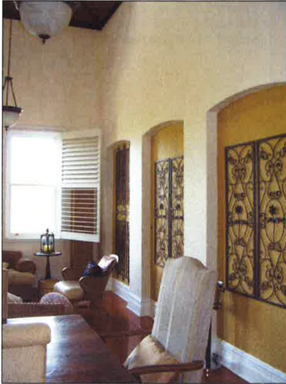
Figure 3.38 The large room also features blind recesses on the northern and southern walls. The walls have been rendered with similar finish to the exterior of the building. The room also retains a high leaded window on the eastern wall (below, top right, corresponding to the stair mid landing).
