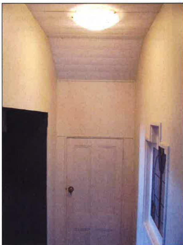
Figure 3.43 The rear landing (first floor of the rear wing) has a timber boarded raked ceiling with small store and modern bathroom at each end. Note the leaded window. The bathroom retains an early timber battened ceiling.
