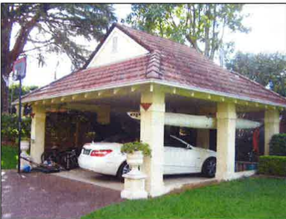
Figure 3.14 The eastern driveway and carport are later additions to the site (c. 1996). The carport has concrete slab floor and gabled hipped roof supported on solid rendered brick columns
