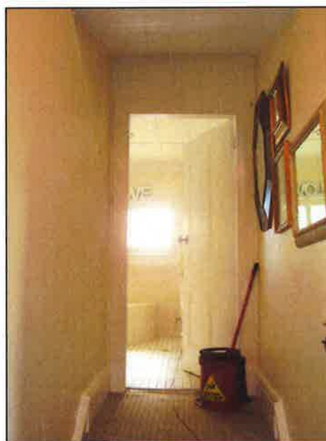
Figure 3.43 The rear landing (first floor of the rear wing) has a timber boarded raked ceiling with small store and modern bathroom at each end. Note the leaded window. The bathroom retains an early timber battened ceiling.
