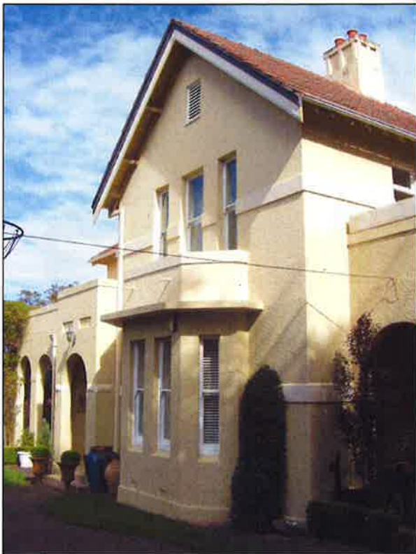
Figure 3.16 The front, eastern façade of the building has a gabled projection with single storey faceted bay, central entry and verandah which wraps around the south eastern corner of the building.
