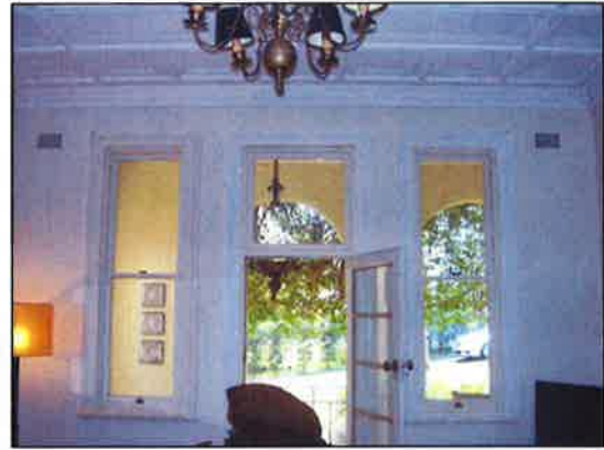
Figure 3.30 The north western room on the ground floor of the main wing retains a high decorative plaster ceiling and original timber joinery. A window has, however, been modified with door added to access the northern verandah.
