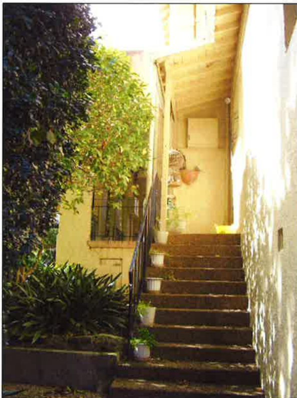
Figure 3.22 A small porch with skillion roof supported on timber posts is located at the northern junction of the main and rear wings. Steps extend down the north western to the garden area.
