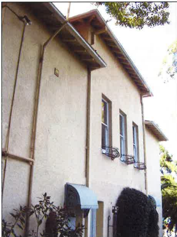
Figure 3.24 The western façade which also has openings to a lower ground area.
