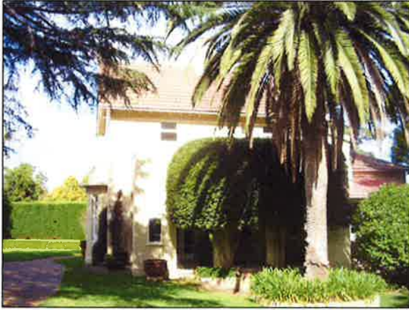
Figure 3.20 The north eastern façade. The verandah has modern ceramic tiled floor and steps down to the northern garden area.
