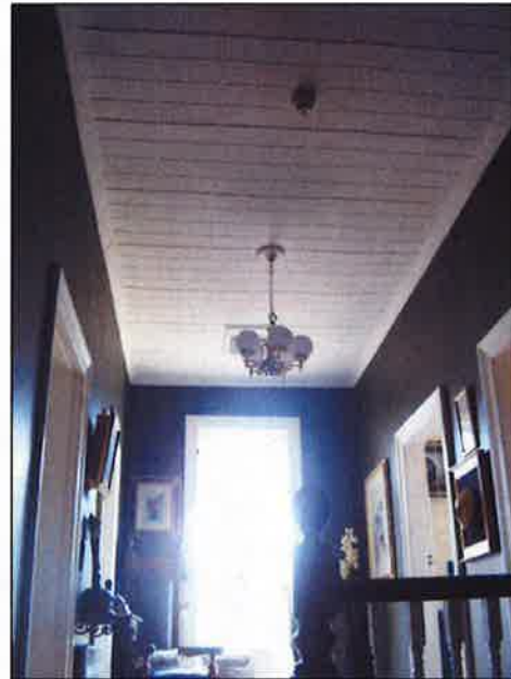
Figure 3.41 A deep window opening on the eastern wall of first floor hallway has been converted into a doorway and accesses the balcony over the front verandah.
