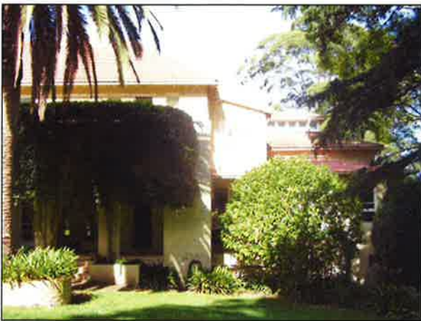
Figure 3.21 The rear wing is stepped back from the main section of the building and has hipped and skillion roof forms clad in ceramic tiles and corrugated steel. The central section of the roof is raised with clerestory windows and hipped roof over.
