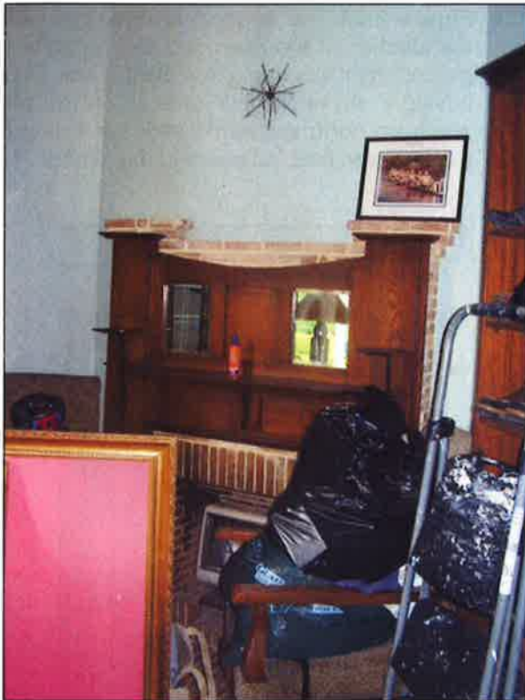
Figure 3.32 The front, south eastern room features a splayed fireplace with timber surround and pressed metal ceiling and timber joinery including timber panelled doors.
