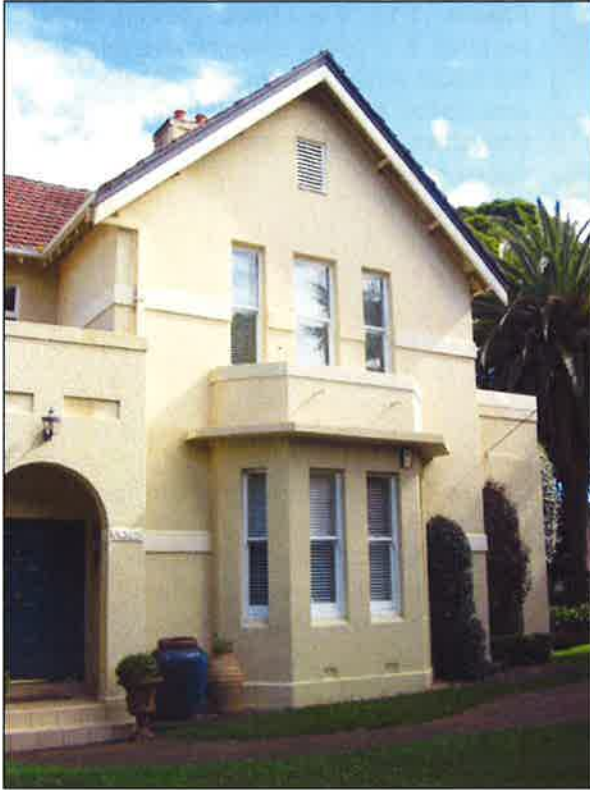
Figure 3.18 The building entry retains the original door opening and sidelights, however the door appears to have been replaced and porch area modified with opening to the verandah infilled and modern tiles added to the floor and steps.
