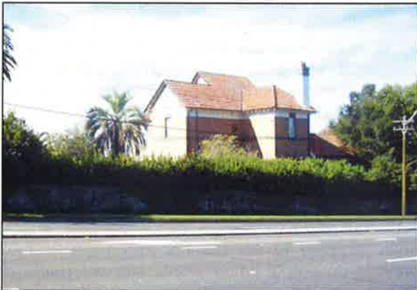
Figure 3.4 No. 67 Mona Vale Road retains its face brick and rough cast rendered walls and chimneys and overall form and character including distinctive roof form and also makes a positive visual contribution to the area.
