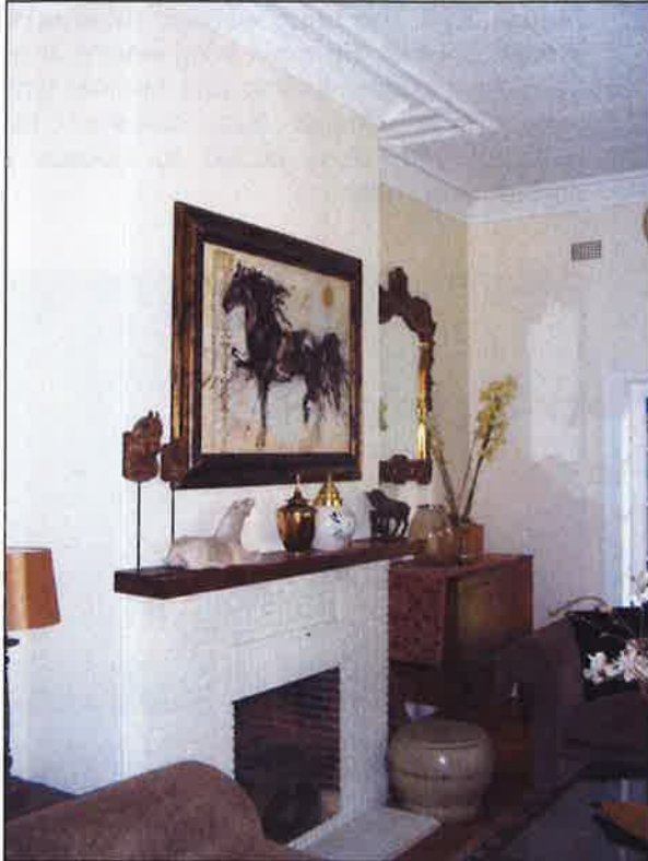
Figure 3.28 The front, north eastern room retains original high pressed metal ceiling and decorative coving and timber joinery and floor. A painted brick fireplace with simple timber mantle located on the western wall appears to have been modified. A photograph dated 1930 ( Figure 2.6 ) shows the original fireplace, marble and timber surround. It would appear that the fireplace was modified as part of the early 1940s works to the building.
