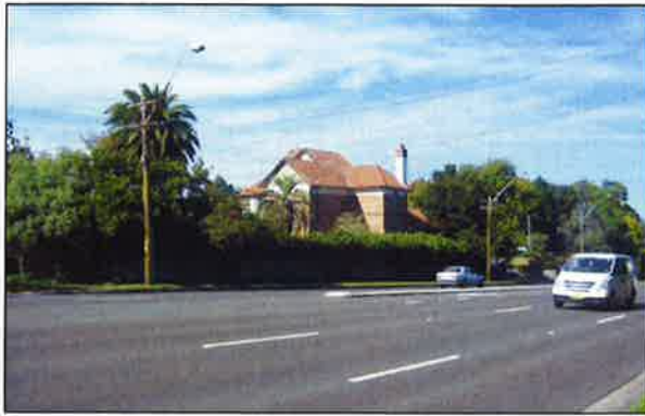
Figure 3.3 Also located diagonally opposite the site, No. 67 Mona Vale Road is also a prominent two storey Federation period dwelling that is also highly visible, particularly when travelling south along the roadway.
