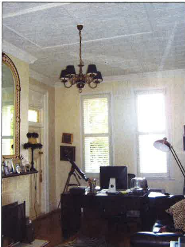
Figure 3.33 The south western room on the ground floor of the main wing has high pressed metal ceilings and original doorway to the front verandah return. The room also has a painted brick fireplace and breast and original timber joinery and windows.
